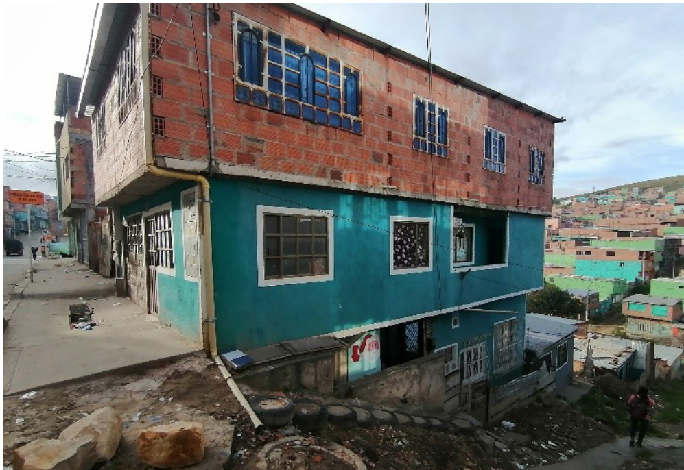
Figure 2: Sloping street in the Caracolí neighborhood. (2022)
