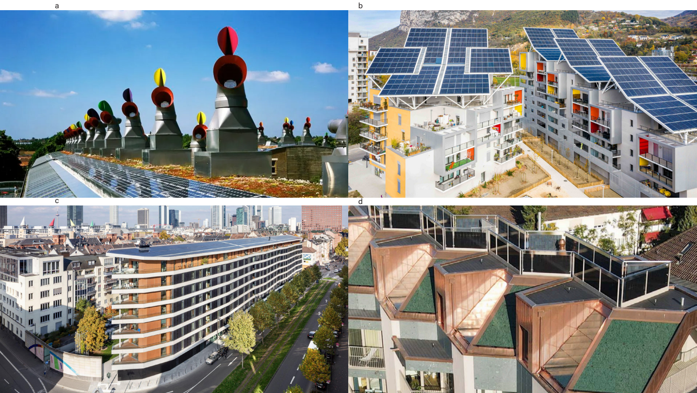
Figure 2: Projects BAPV (a,b) and BIPV (c,d) a) BedZED, London, 1999-2002. b) ABC, Grenoble, 2020. c) Aktiv Stadhaus, Frankfurt, 2015. d) Apartment building, Zurich, 2022 a) Twinn (2003); b) France Villes & Territoires Durables (2023); c) Shūco (2023); d) Megasol (2021)
