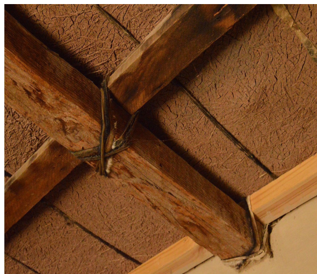
Figure 4: Caruna tied with cowhide. Gunwales and struts made of rough pine wood. Source: Own work
