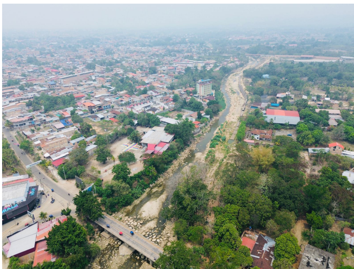
Figure 5. Aerial view of the area surrounding the Cumbaza Bridge (2024). Source: Author's own work (2024)
